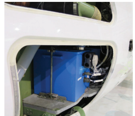
Installation of (2) TB44 Certified Lithium-ion Batteries in DHC-8-200 aircraft
